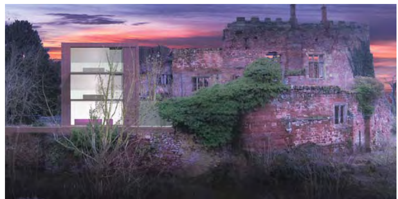
A New House in a Ruined Castle, Astley Castle, Warwickshire
