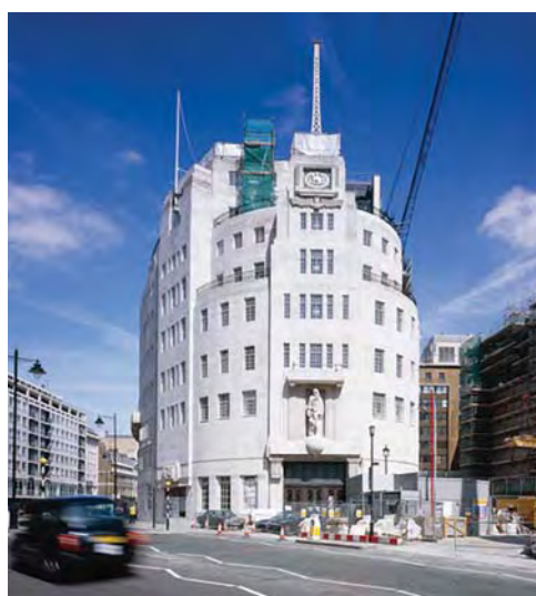
Conservation and Refurbishment of Broadcasting House
